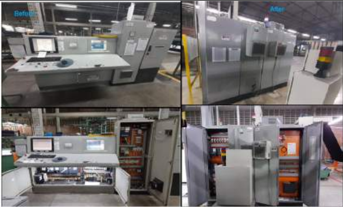
Figure 5: Panel before and after retrofitting.
