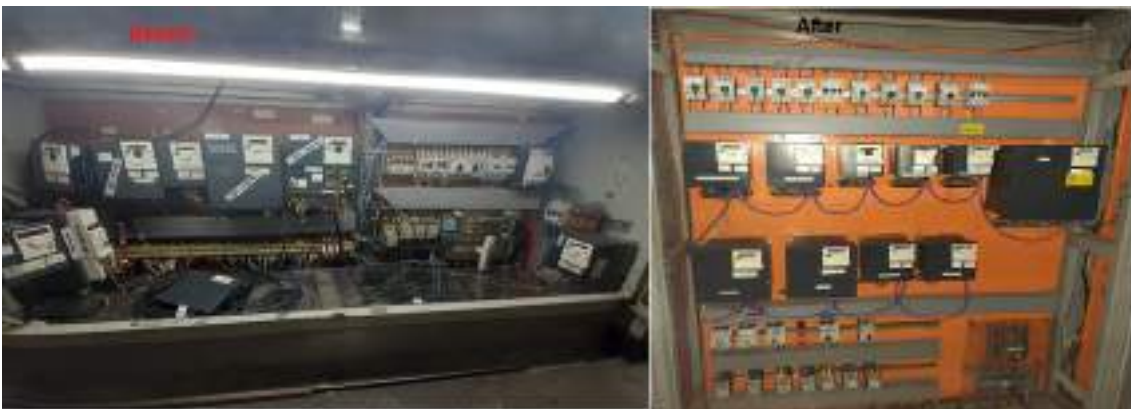
Figure 6: Fixing frequency converters before and after retrofitting.
