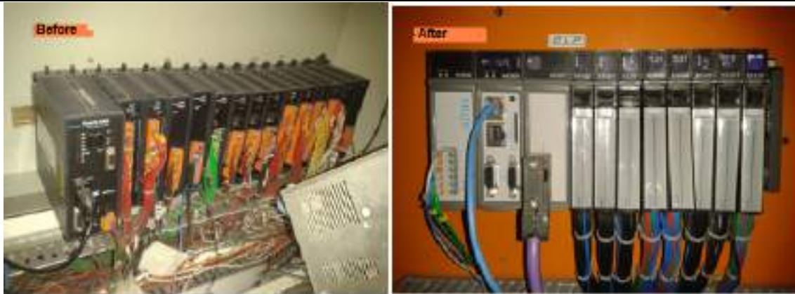
Figure 7: Fixing the PLC before and after retrofitting.
